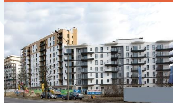
Residential Park, Bielany – etape 2
