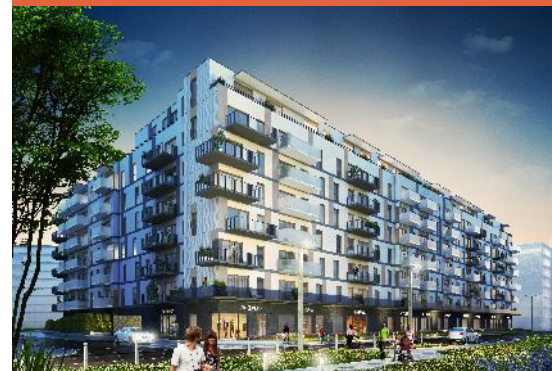
Residential Park, Bielany – etape 3
